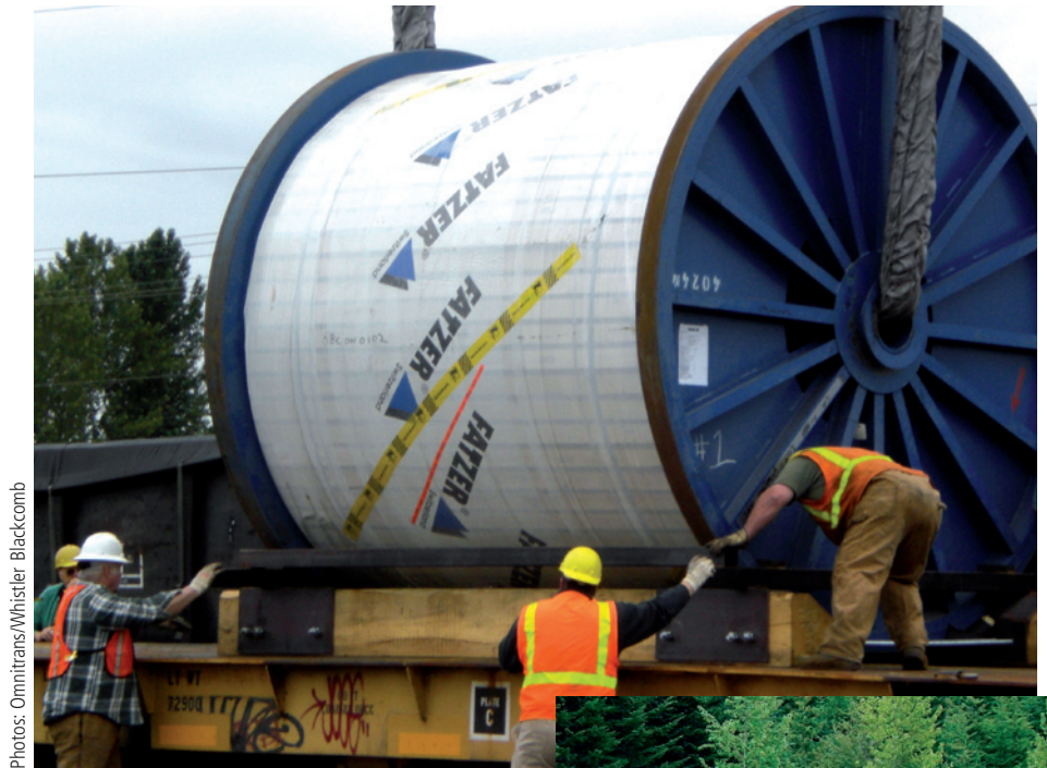
Coils of steel rope on their way to the construction site of a record-breaking aerial tramway in Whistler Mountain (Canada).
